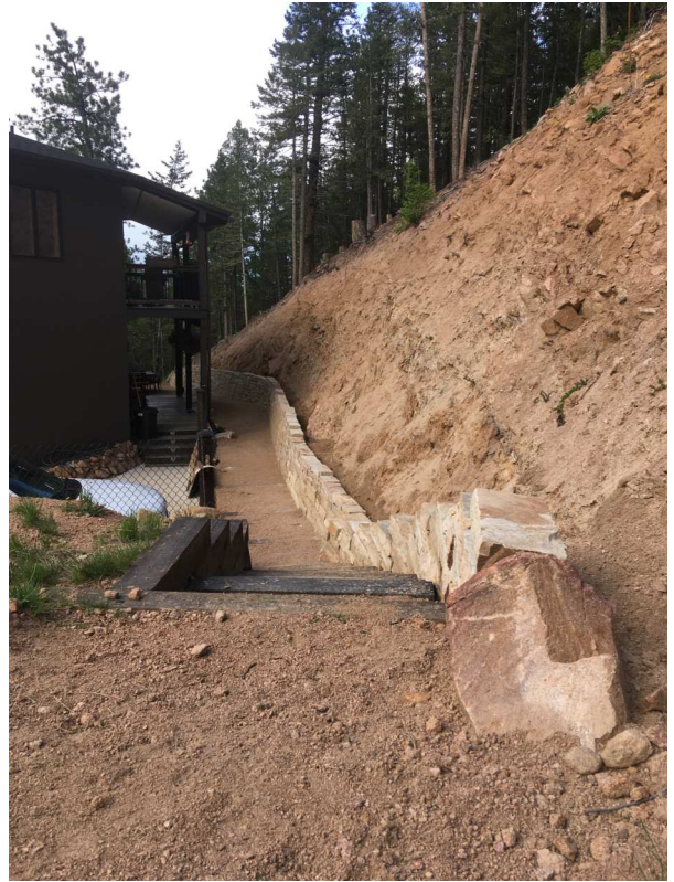
80 foot retaining wall
