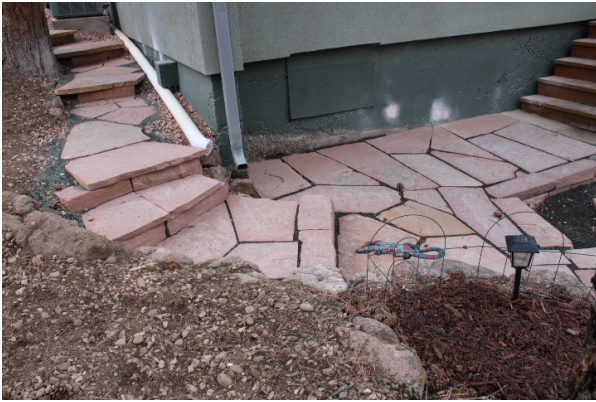
steps and walkways
