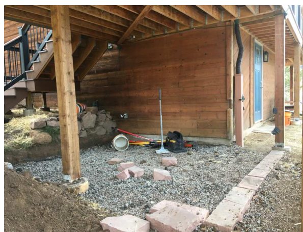
foundation for square patio with block border
