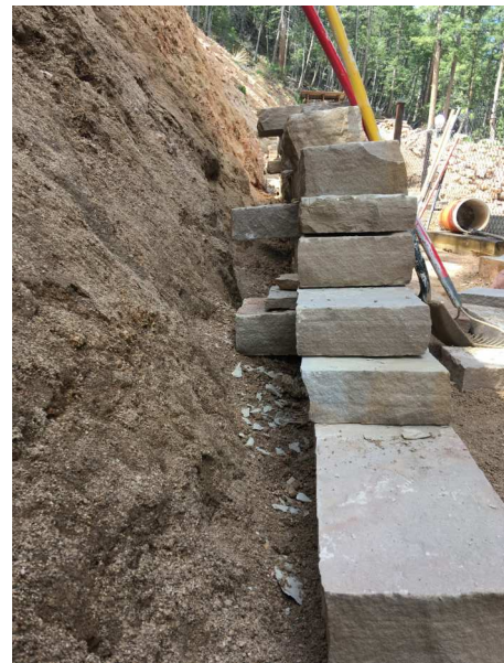
retaining wall tiebacks
