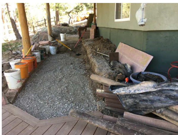
foundation for path and retaining wall
