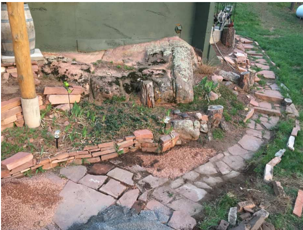
foundation for path extension
