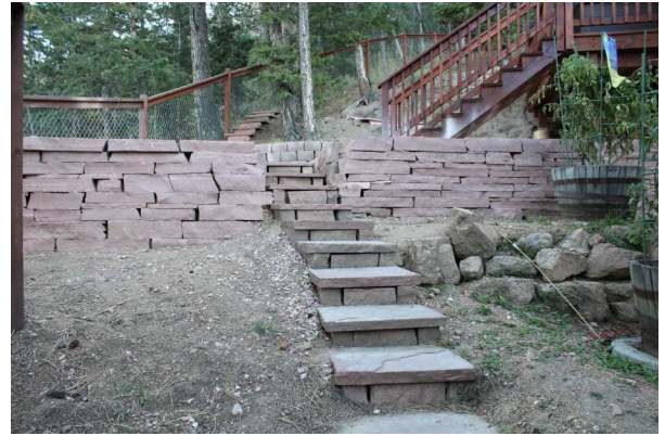
steps to patio behind retaining wall
