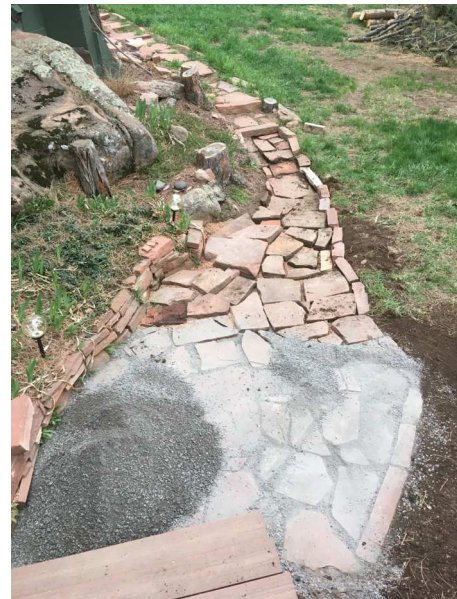
setting and filling gaps
