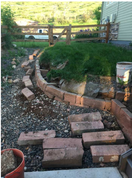
garden wall with tiebacks
